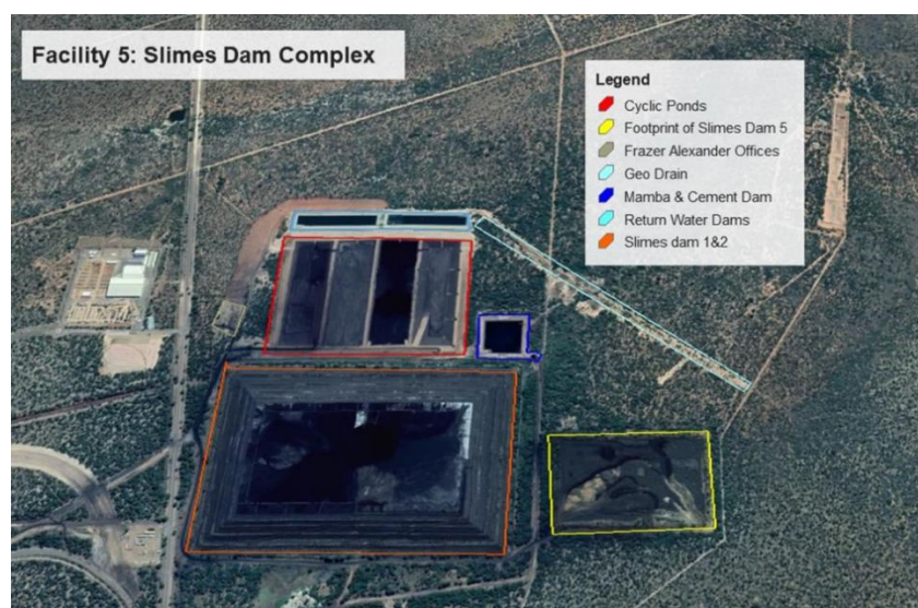
Figure 2.8 Facility 5 - Slimes Dam Complex
