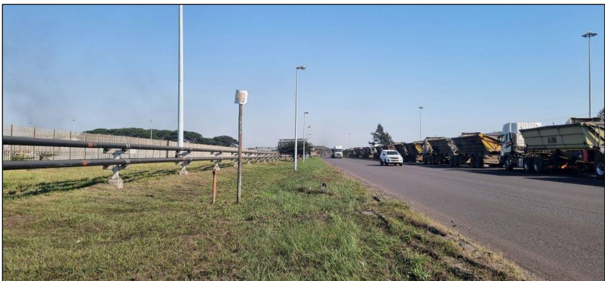
Plate 3: Photograph showing the proposed transmission line route which follows existing roads within the Port.
