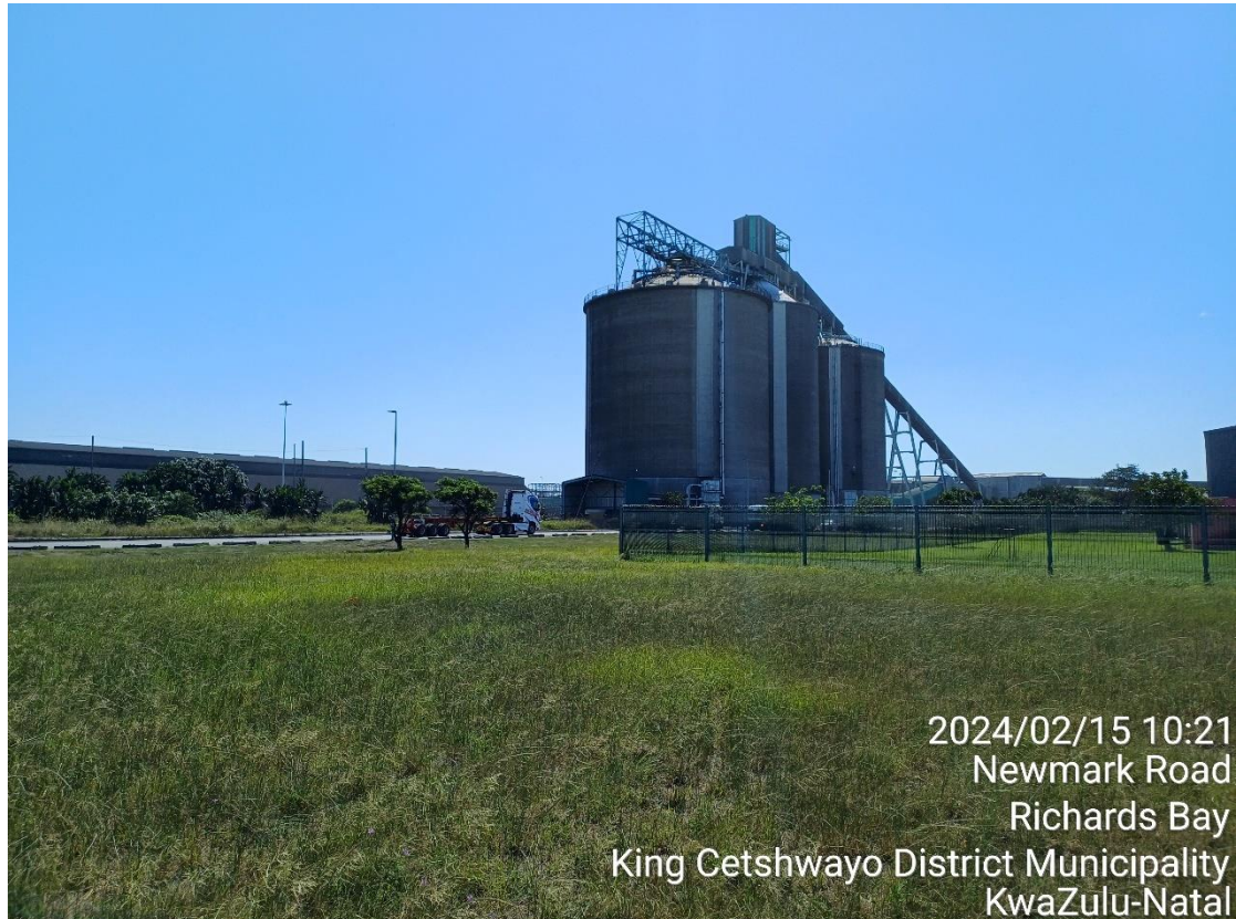
Figure 5-1: Current silo's situated opposite to the proposed generator complex site.
