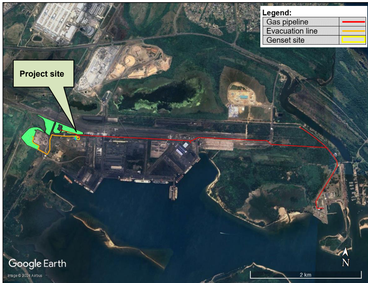
Figure 11-4: Location and extent of the Transformed Alluvial Grassland vegetation type associated with the project site
