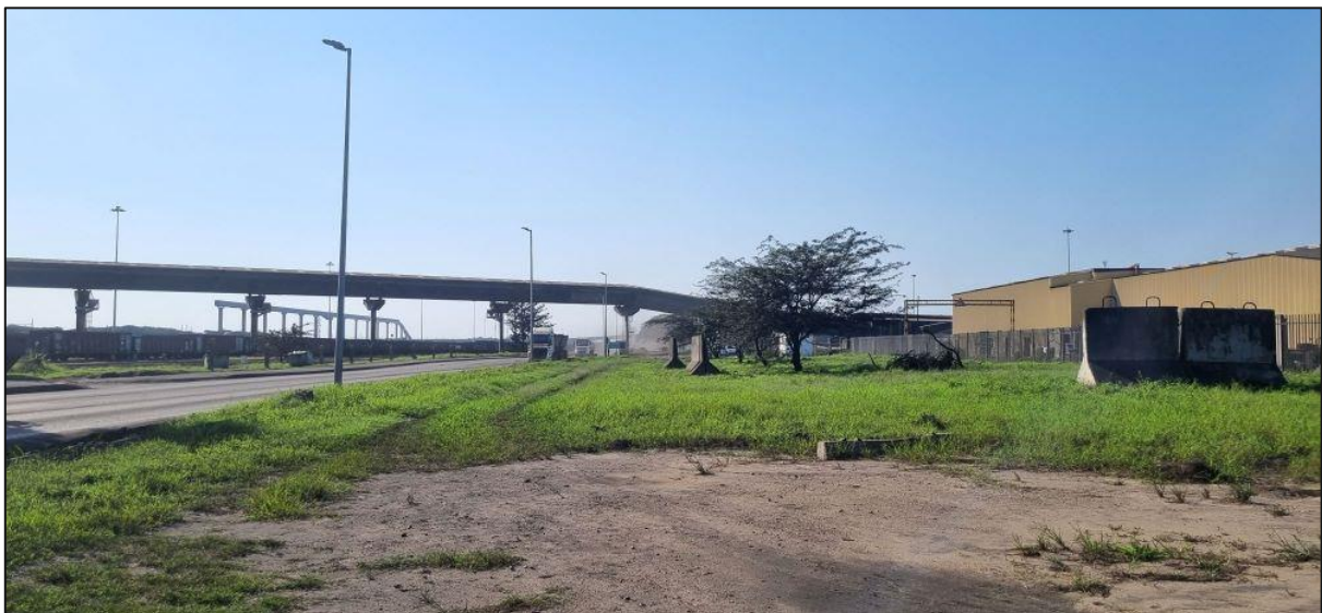
Plate 2: Photograph showing the proposed transmission line route on the central portion of the project site.
