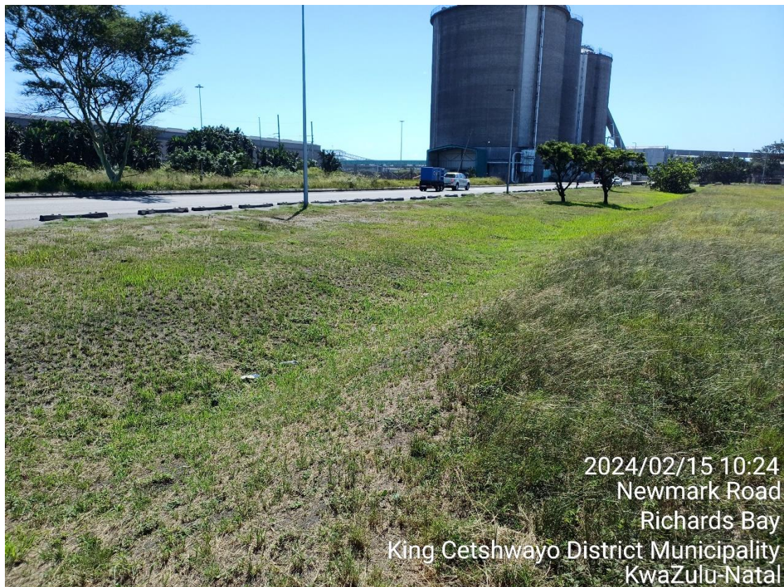
Figure 6-9: Silos located opposite the generator project area.
