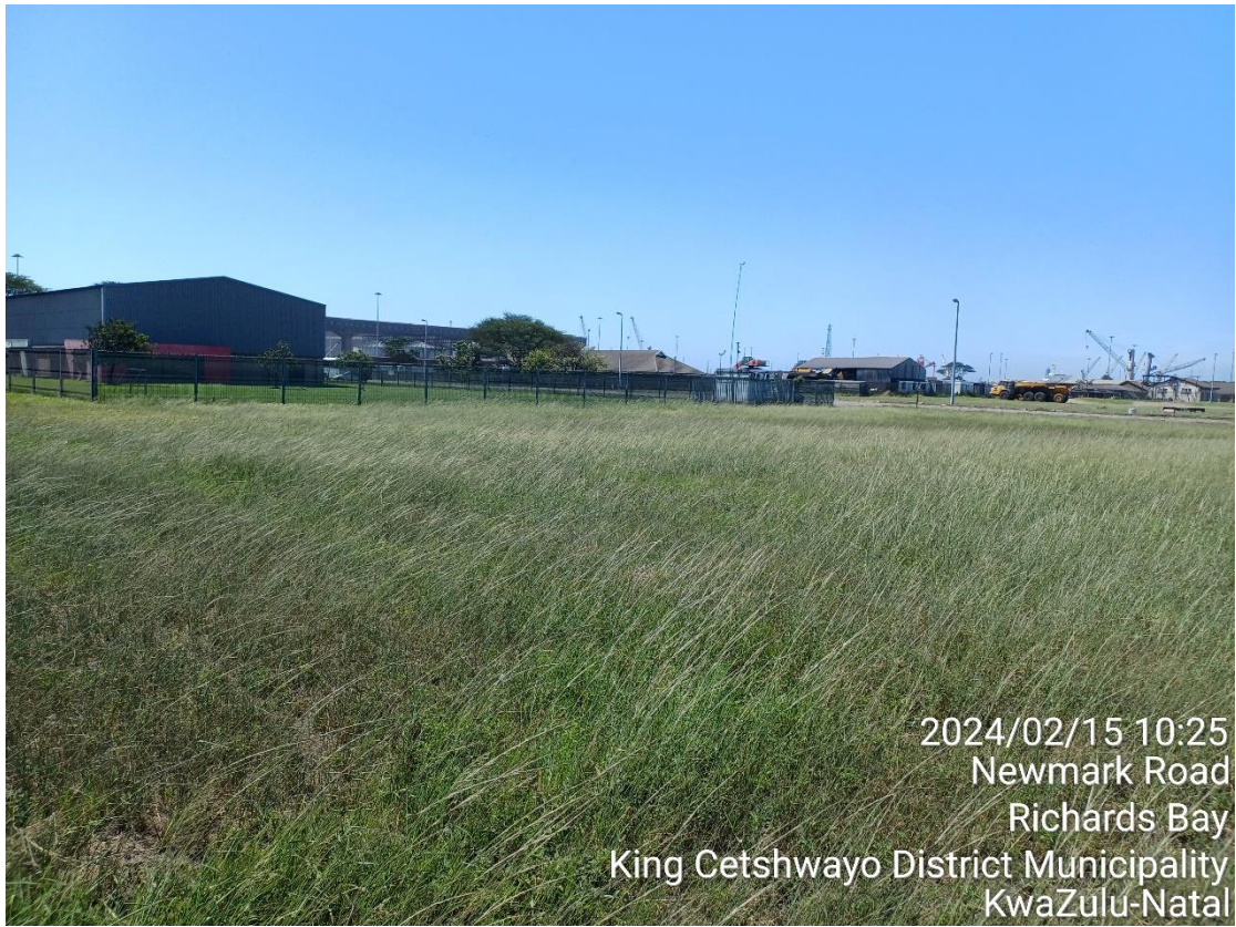
Figure 6-10: Buildings located next to the generator project site.
