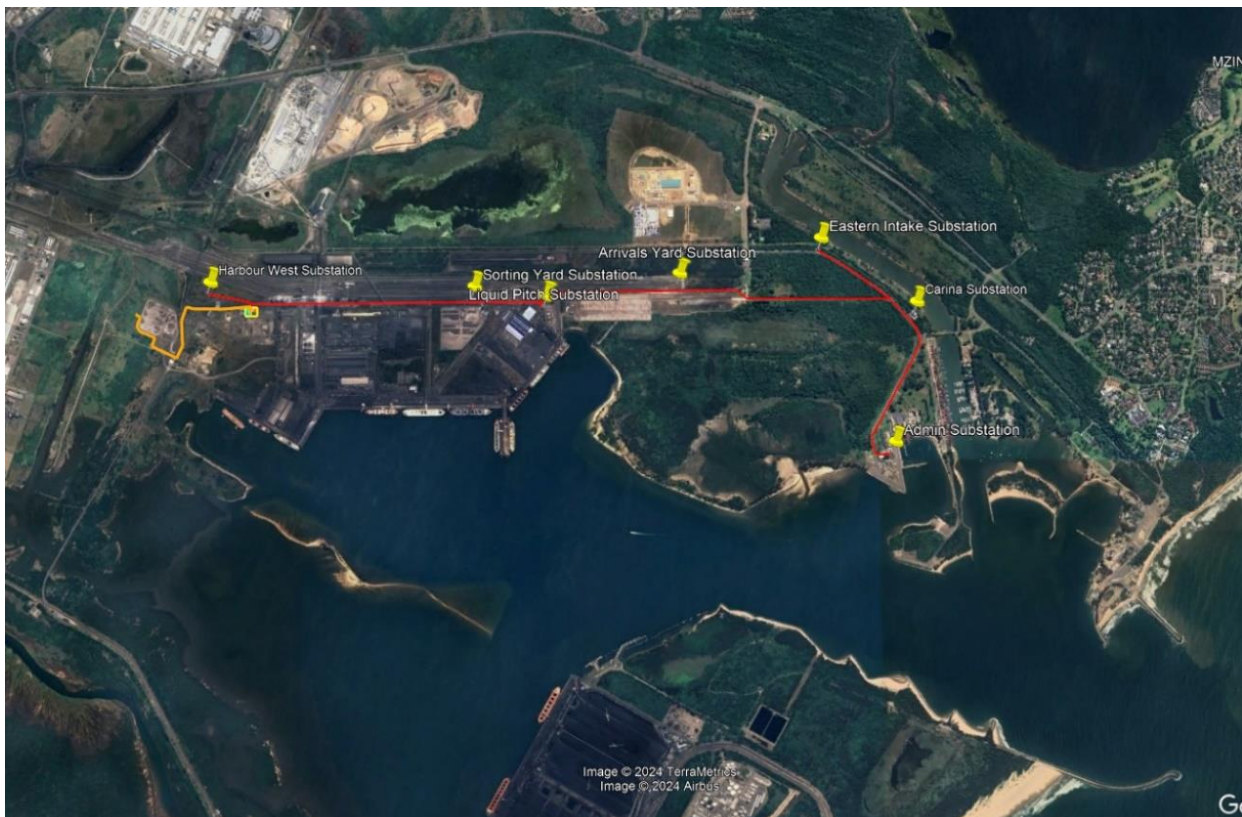
Figure 11: Current aerial imagery from 2024
