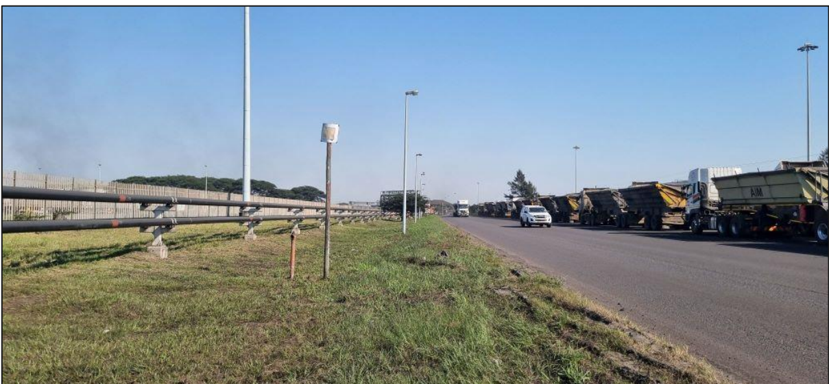
Plate 3: Photograph showing the proposed transmission line route which follows existing roads within the Port.
