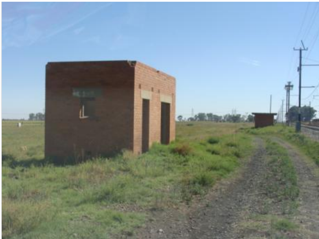
Figure 4-7: Station buildings at site no. 2
