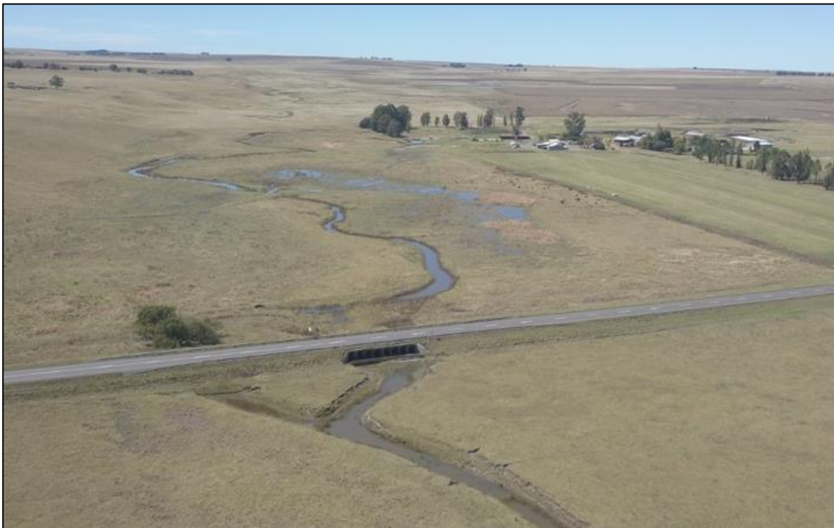
Plate 11-5: Aerial view of the road and culvert crossing through the Channelled Valley Bottom
