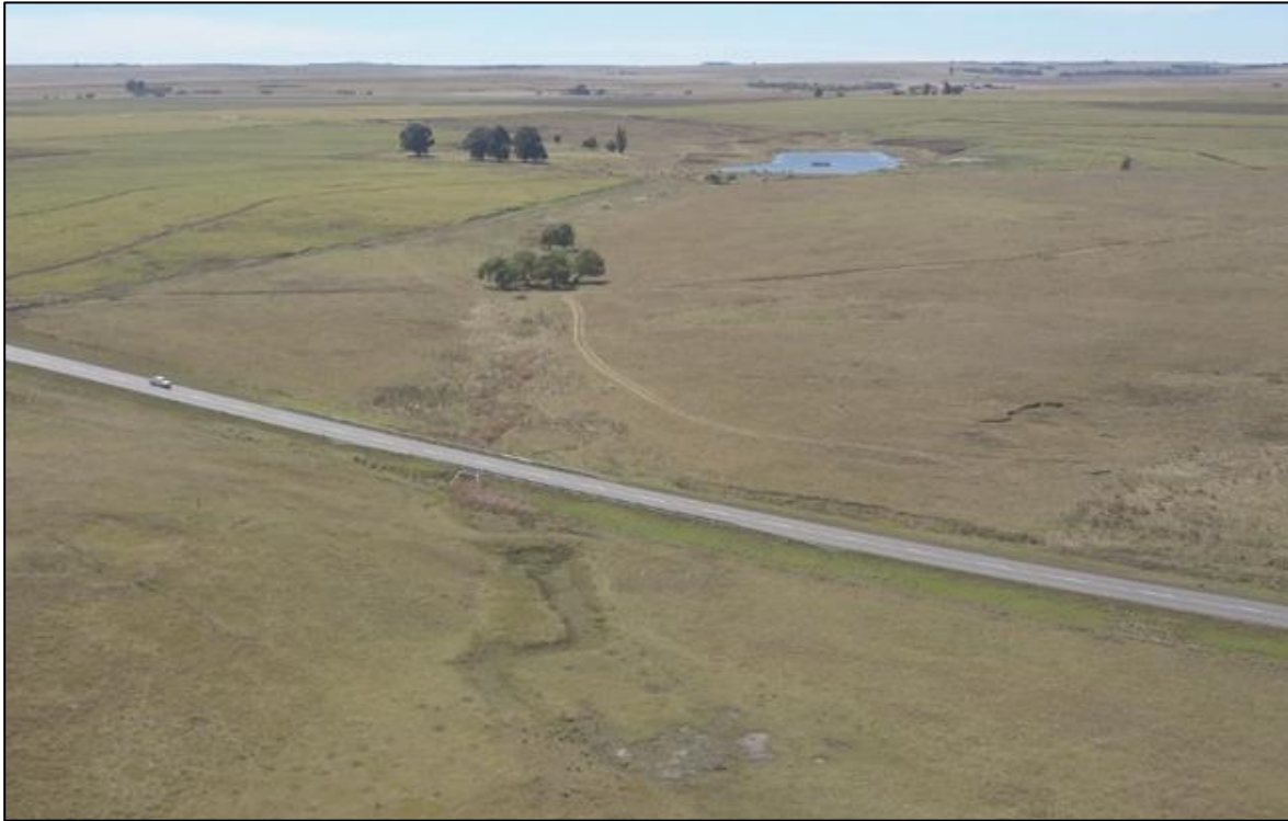
Plate 11-6: Aerial view of the culvert and road crossing the Seep as well as the dam and impoundment area
