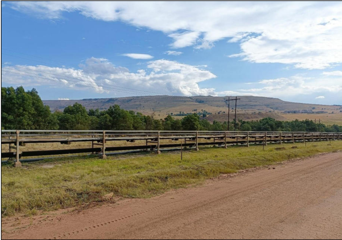
Plate 9-3: View of the mine access road and conveyor system associated with the mining operations
