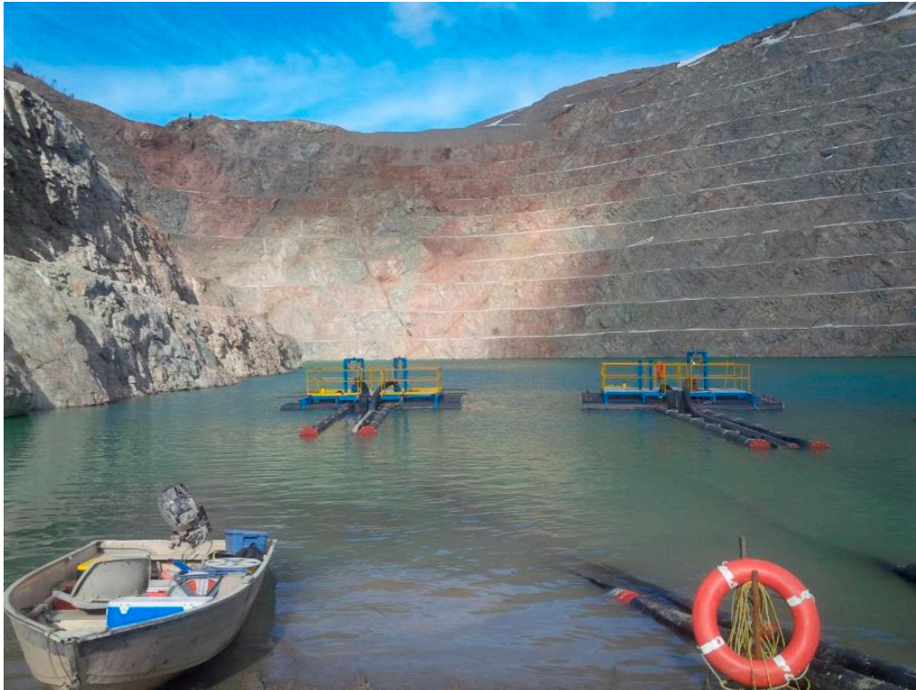
Figure 8. Springer Pit Lake and dewatering infrastructure at Mount Polley Mine, BC, Canada.
