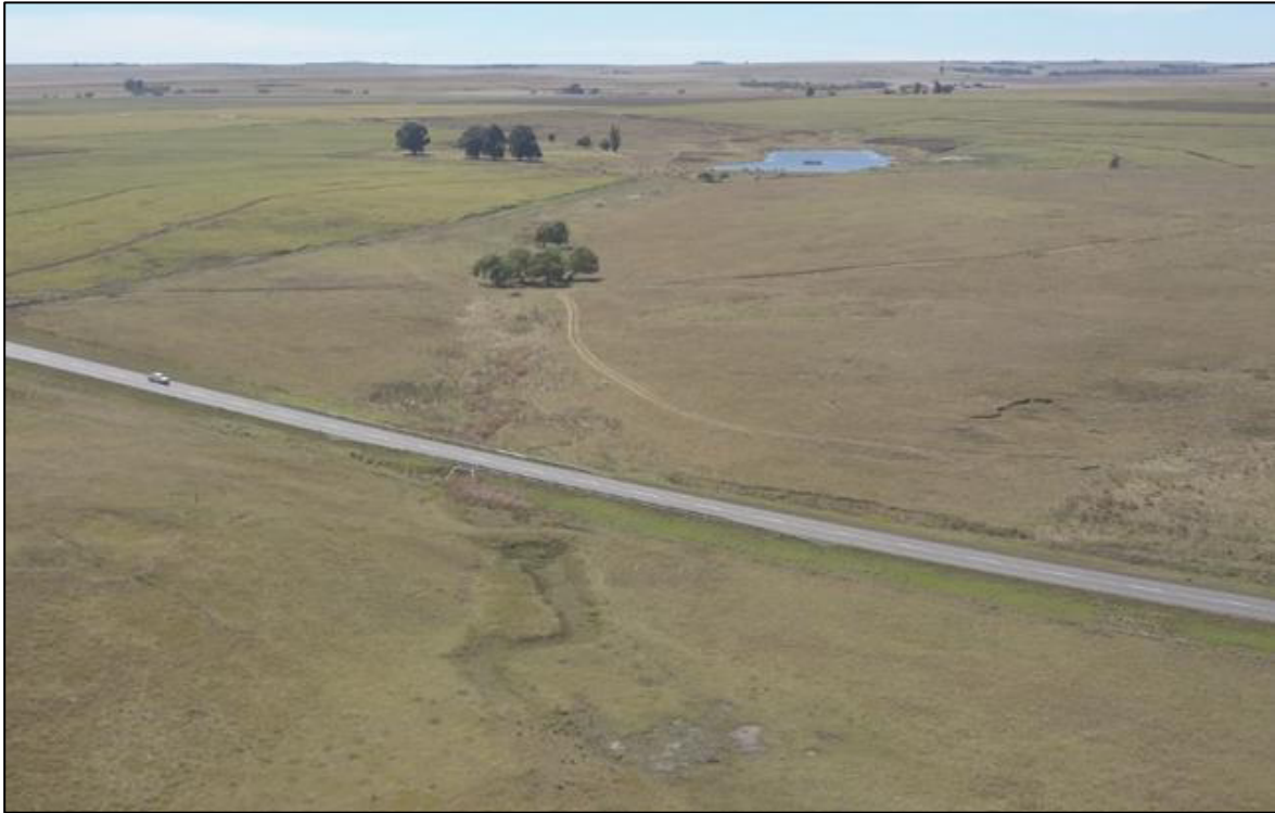
Plate 11-6: Aerial view of the culvert and road crossing the Seep as well as the dam and impoundment area
