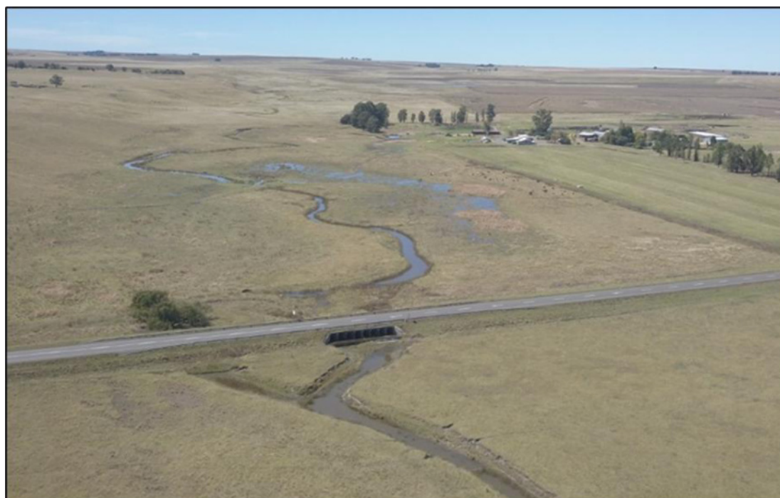
Figure 5-3: Aerial view of the road and culvert crossing through the Channelled Valley Bottom
