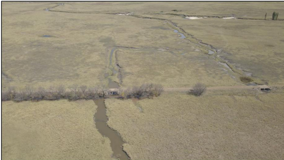
Figure 5-5: Aerial view of the railway and culvert crossings in the Flood Plain as well as the canalised water flow
