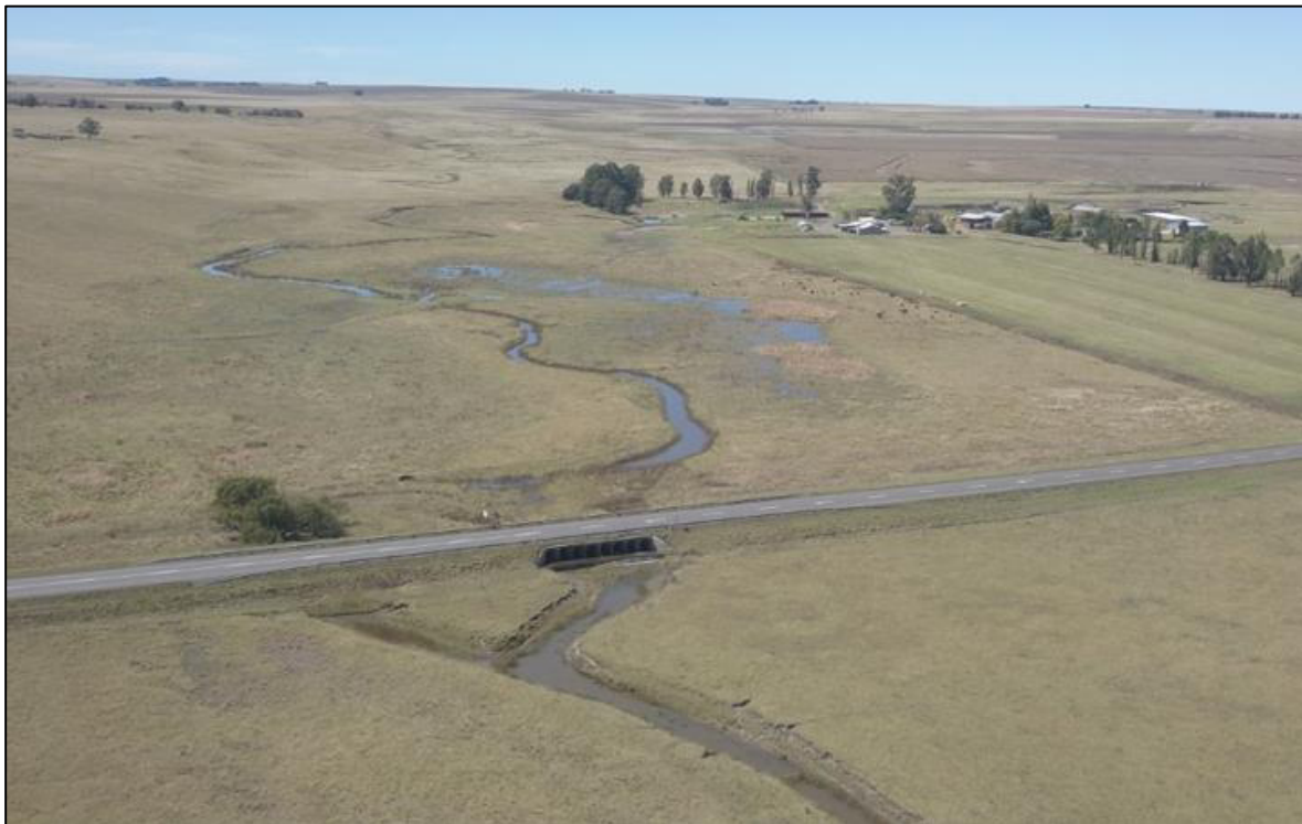
Plate 11-5: Aerial view of the road and culvert crossing through the Channelled Valley Bottom
