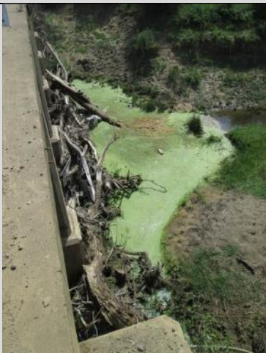
Bridge impeding flow and debris build up
