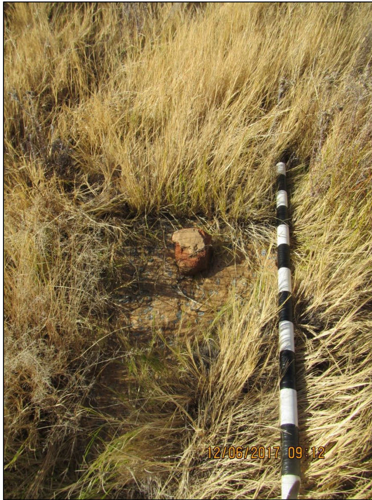
Figure 16 – View of concrete foundation and brick with mortar at Site 002. Scale in 10cm increments.
