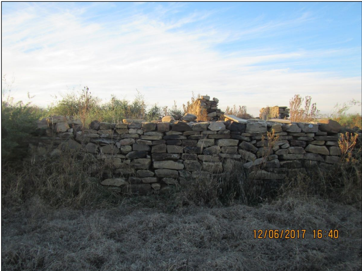
Figure 50 - Sandstone structure, Site 013f.
