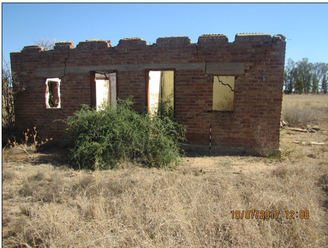
Figure 97 – Rear view of the same building. The steel doorframes can be seen.
