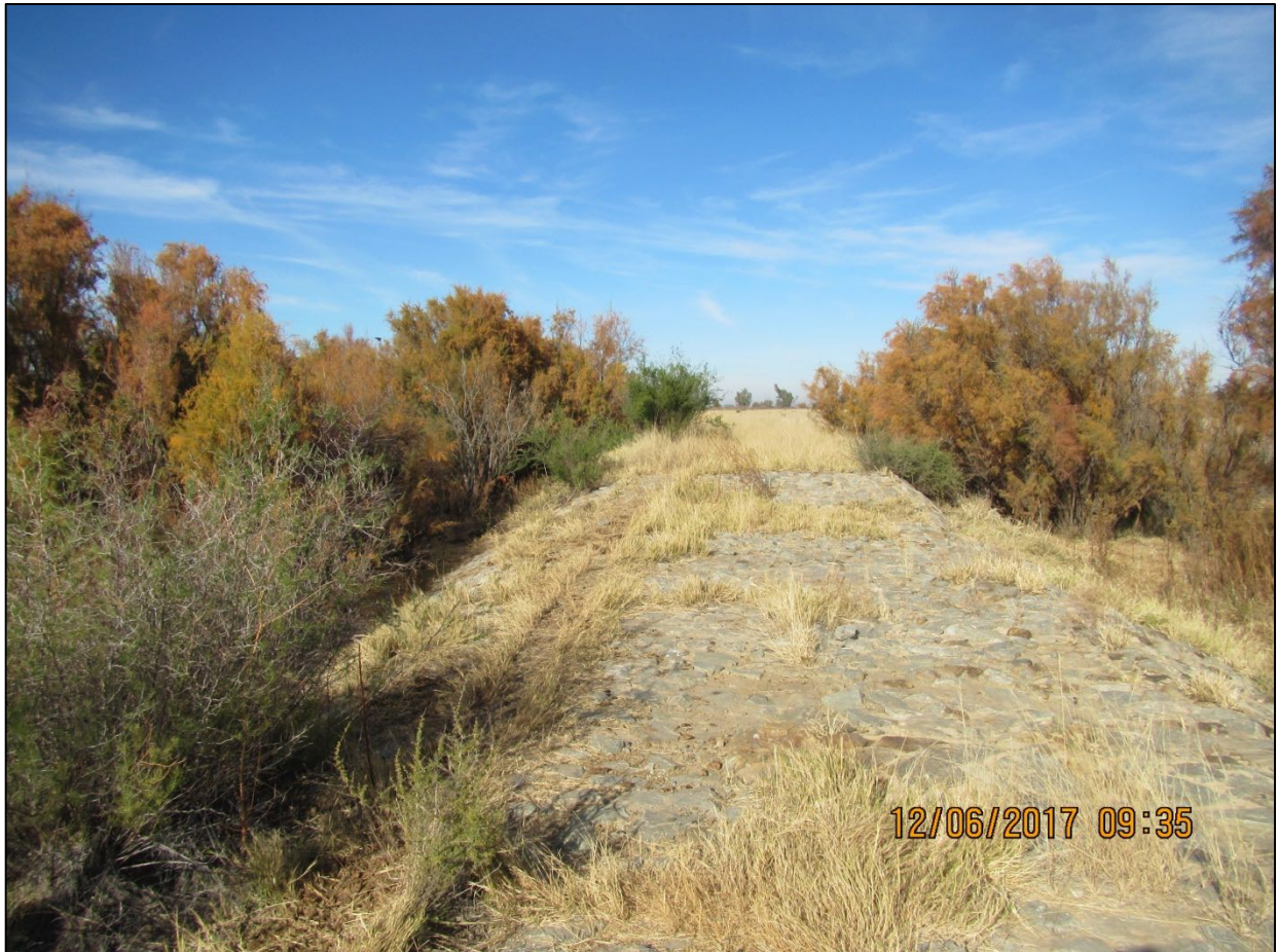
Figure 19 - View of the stone-packed spillway of the dam at Site 003.
