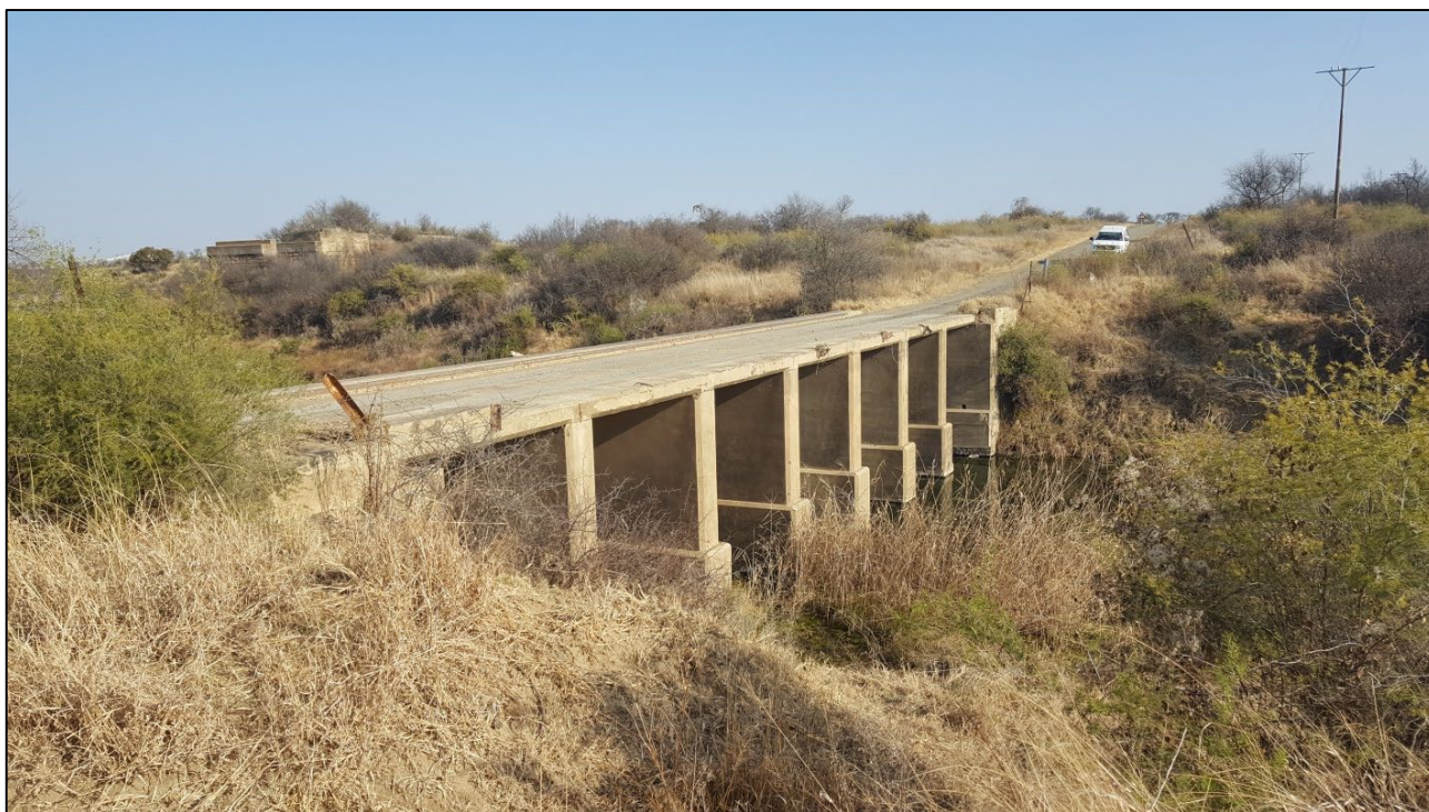
Figure 95 – General view of the concrete road bridge at Site 33b.
