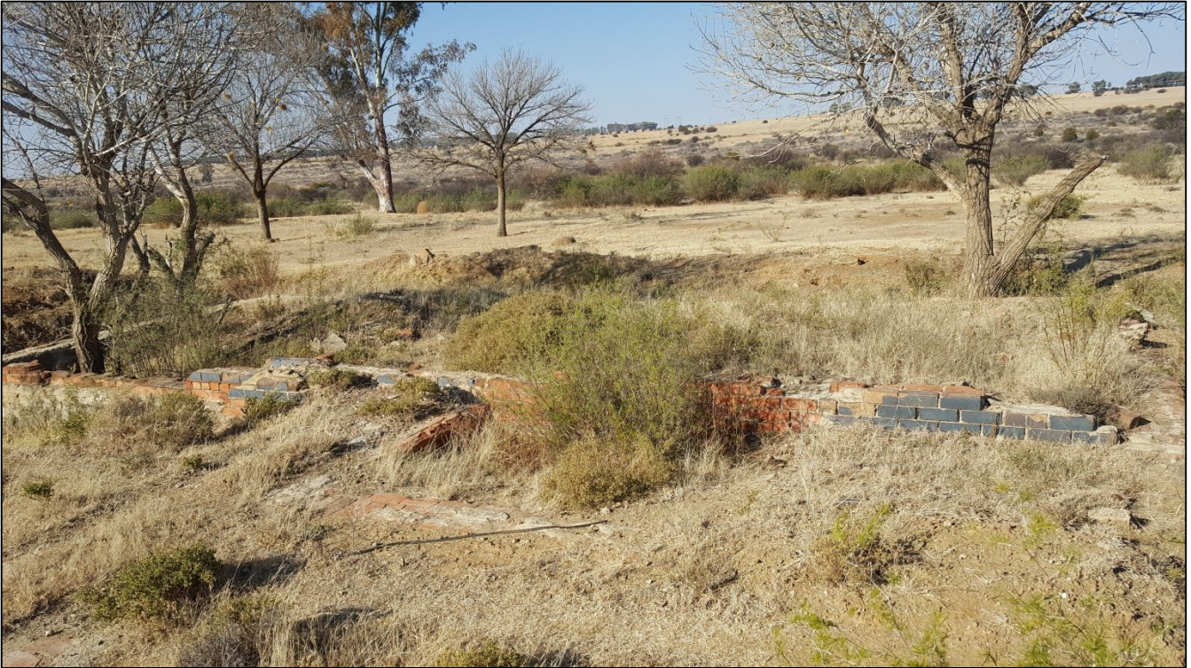
Figure 73 - The foundation remains of the outbuilding at site 023
