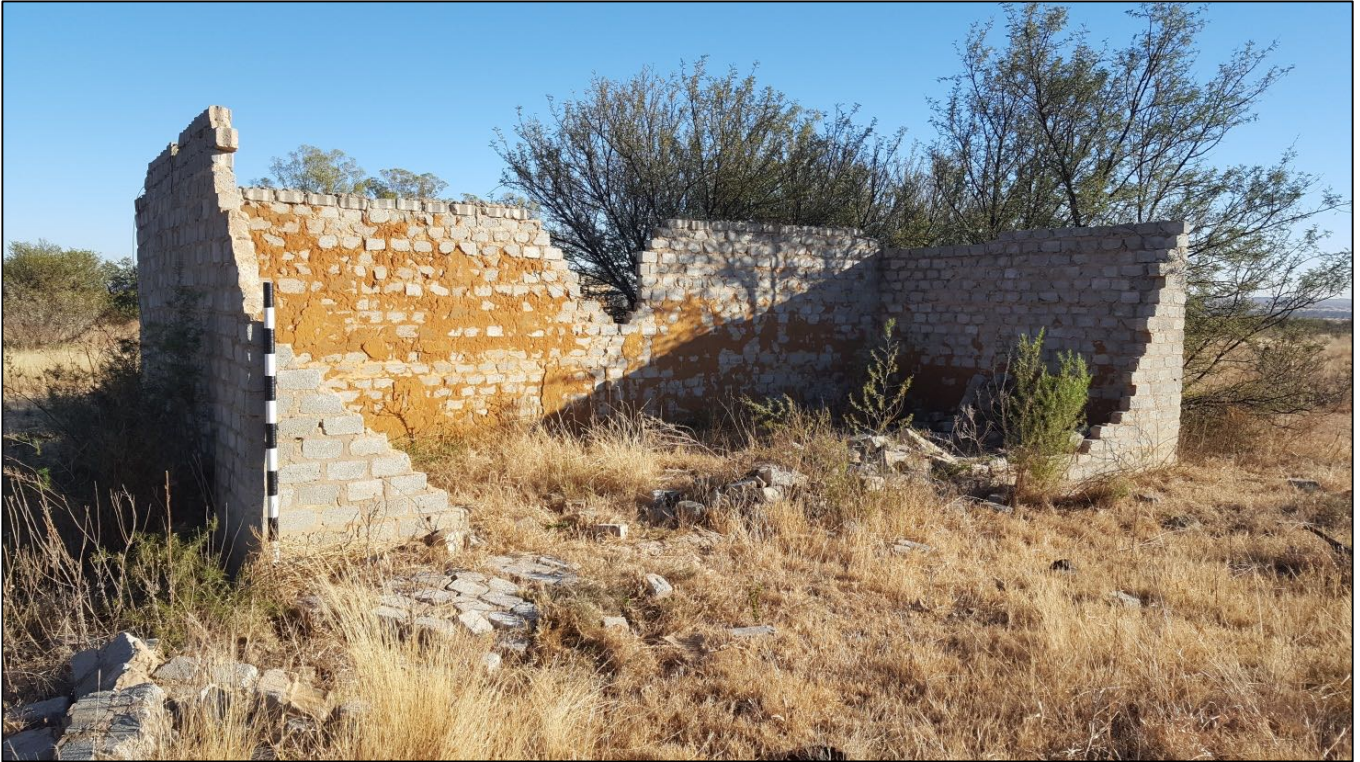
Figure 54 - Cement brick structure at Site 015a.
