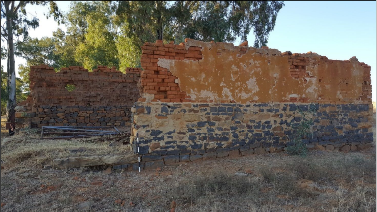
Figure 77 – View of the wagon shed, Site 025. Scale is in 10cm increments
