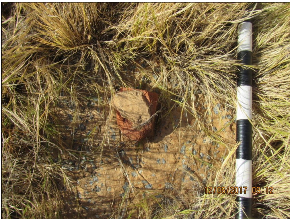
Figure 17 – Closer view of concrete foundation and brick with mortar at Site 002. Scale is in 10cm increments.
