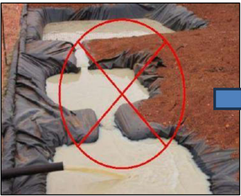
Figure 2: Historical industry practice of Drill sump vs Sediment Reduction Unit.
